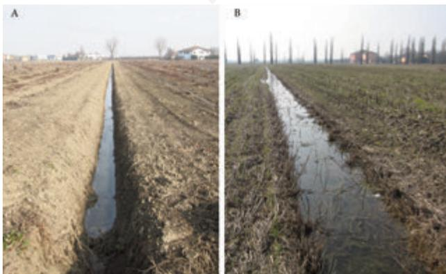
Figure 2. The Standard 1.1c commits to the maintenance of the farm channel network. (A) channel maintained properly and (B) channel invaded by herbaceous vegetation which does not ensure an effective drainage of water from the fields.
